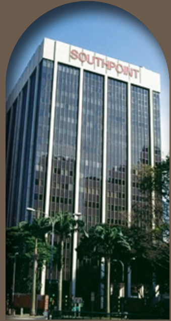
SOUTHPOINT BUILDING (SINGAPORE)
